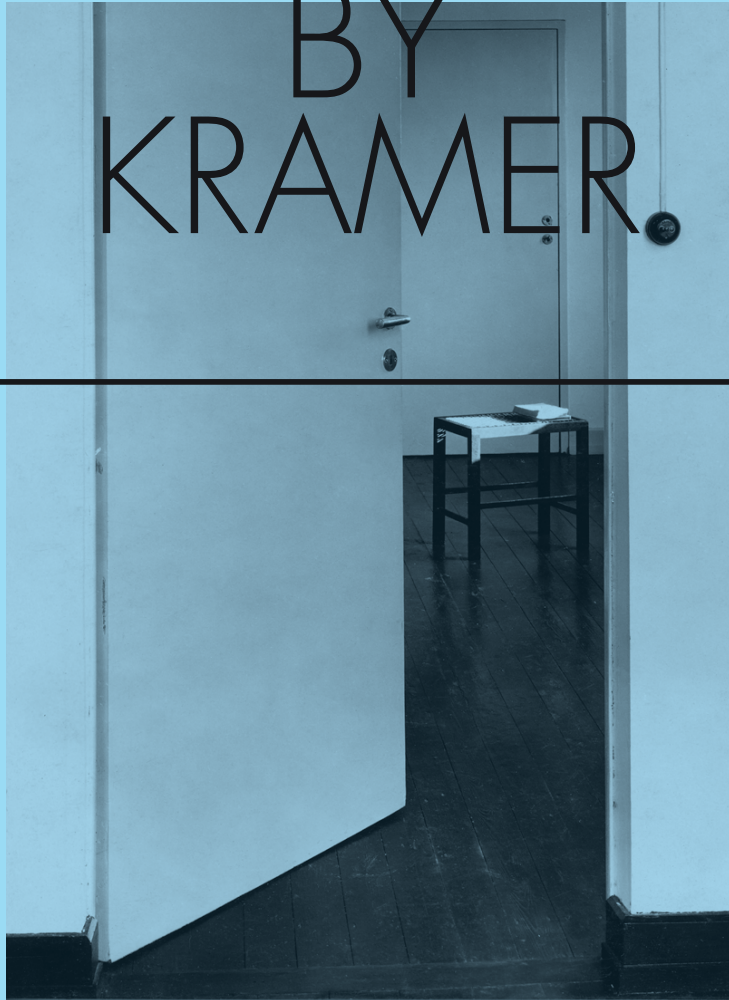
Standard model of plywood door with steel frame PHOTO: H. COLLISCHONN, 1925
