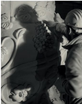
Assistenza in cantiere / On-site assistance
