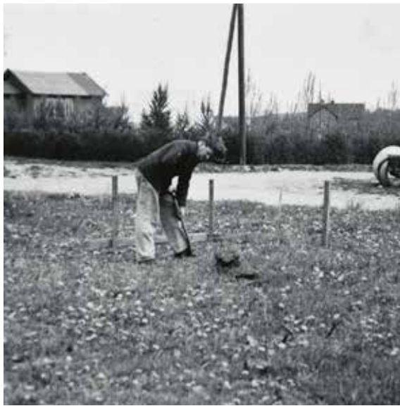
Ejnar Pedersen digs the foundations of PP Møbler.
